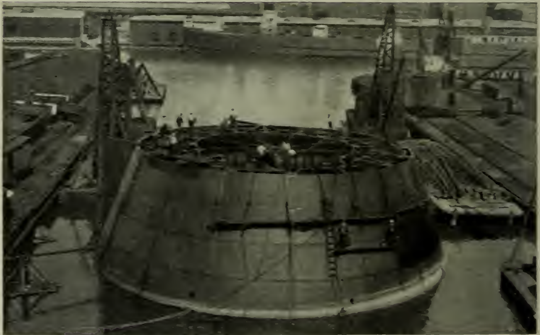
Steel Shell of Wilson Avenue Crib nearly completed.
